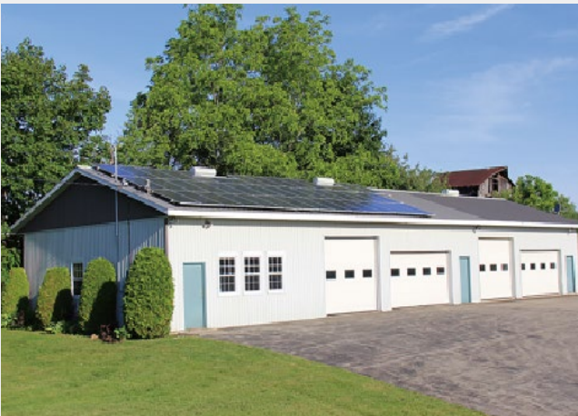
13.2kW Rooftop PV Station in Burlington, Canada
