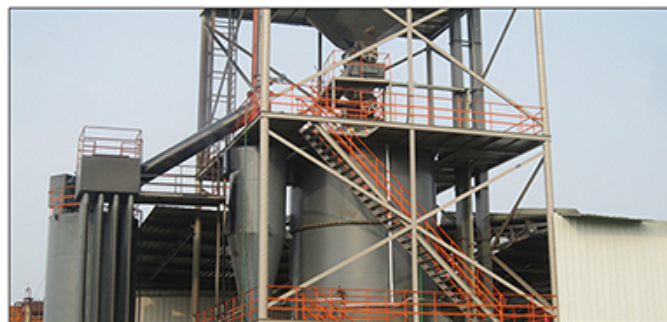
2MW UFBG POWER PLANT
