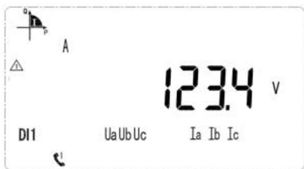
Voltage on A phase is 123.4V
