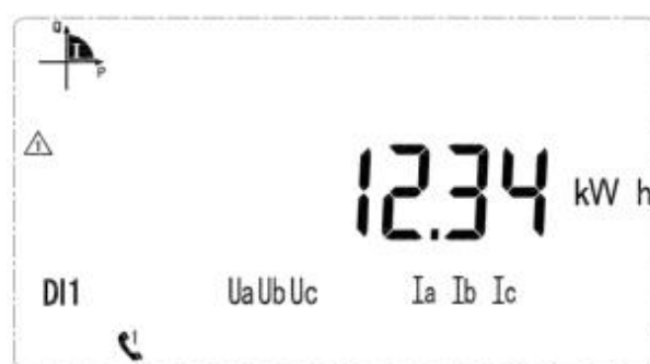
Current reversing active energy 12.34kWh
